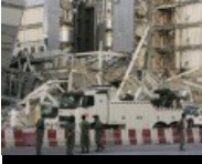
Six-storey building collapses in Deira >>More GN TV video
